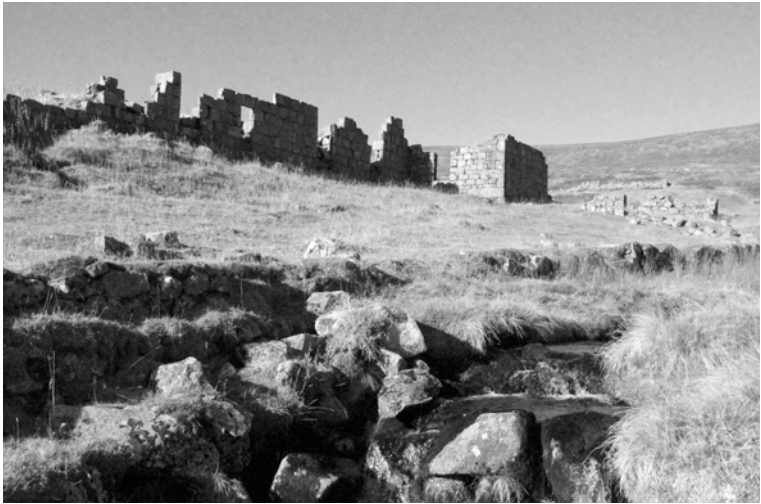
Figure 11. Corrou Old Lodge from the south-east. (October 2010)
