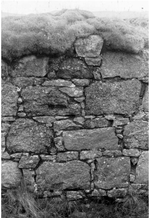
Figure 3. Detail of wall construction (north wall, north range).
