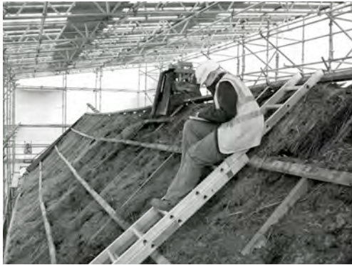
Figure 3. The roof exposed and recording underway.
