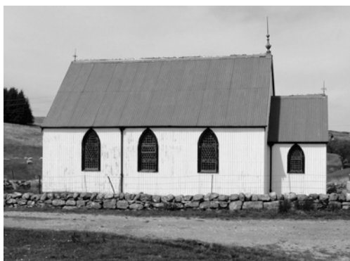
Figures 7 and 8. Dalswinton Barony Church, Dumfries and Galloway (above; 1881) and Syre Church, Sutherland (below; 1891) provide fine examples of the decorative qualities of early tin tabernacles. Syre has lost most of its decorative ridge brattishing, but retains leaded 'gothic'-style windows. (Dalswinton image reproduced under Creative Commons Licence, author Rosser 1954)
