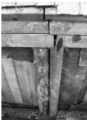
Figure 4 (right). The exposed timber frame at the eaves showing the junction of the 1876 and 1885 construction of the church.
