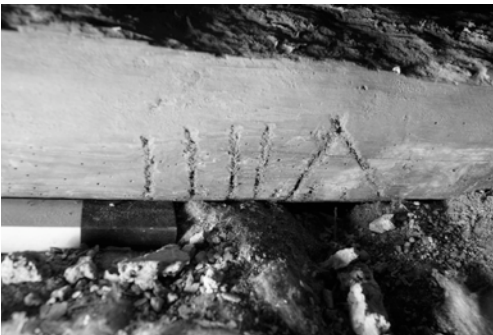
Figure 5. An example of the masons' marks found on the rafters and collars. (© National Trust for Scotland)
