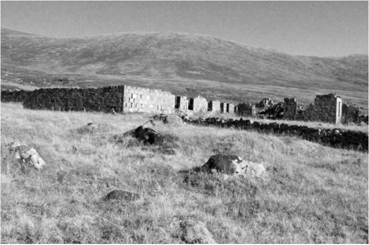
Figure 2. Corroual Old Lodge from the west (October 2010).
