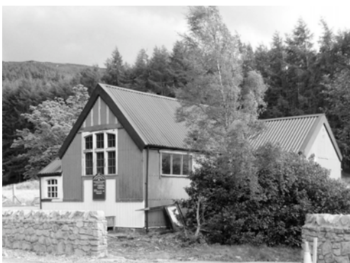
Figure 9. Kinlochewe Church, Highland, a typical example of a Speirs & Co church with a tripartite segmental window and timber boarding detail, very much contemporary with the architectural style at the turn of the 20th century.
