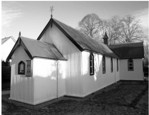
Figure 1. St Fillan's Episcopal Church, Killin after repair in 2011.
