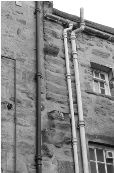
Figure 2. Skews on the building's rear elevation may be remnants of the now demolished backland structures or evidence of the buildings once having a considerably lower roofline. (© National Trust for Scotland)
